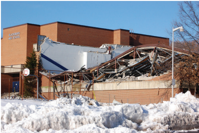
Figure 2.5 Blacksburg, Virginia, High School gymnasium roof after it collapsed under snow load
