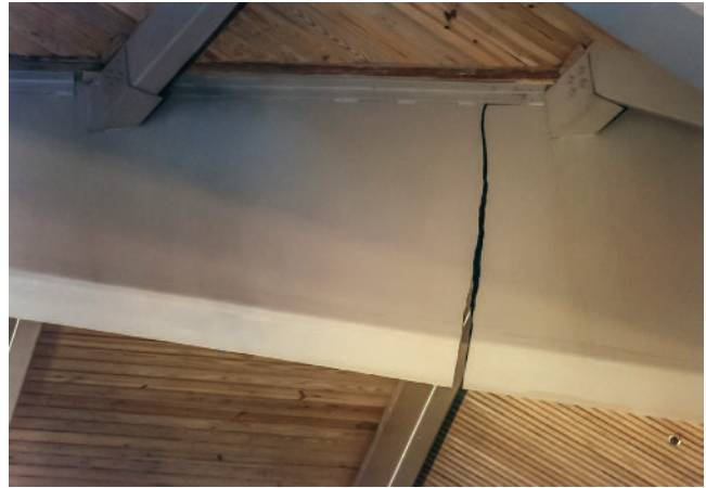
Figure 3.11 Brittle fracture of a steel beam
