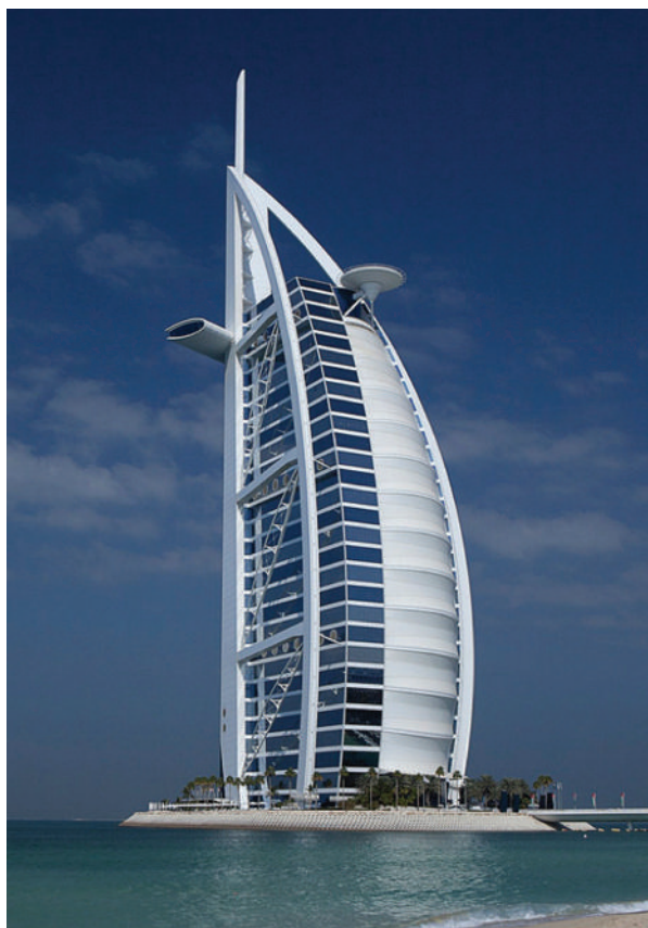
FIGURE 1.1 The Burj Al Arab hotel in Dubai, UAE, is a stunning example of expressed structure in architecture. The steel exoskeleton provides for lateral stability in the region's high winds and perfectly compliments the sail-like shape of the design.
