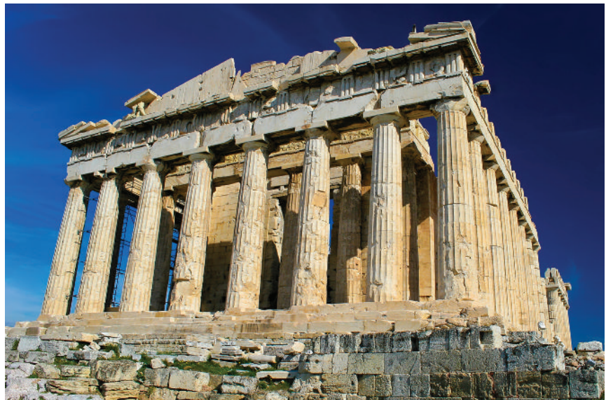
FIGURE 1.3 The Parthenon in Athens, Greece. This most majestic of all ancient buildings—an acknowledged architectural masterpiece—is nonetheless “incorrect” from a purely structural viewpoint. Stone as a building material is weak in tension and unsuited for spanning long distances; hence, the column spacing must be quite close to keep the stone spans very short.
