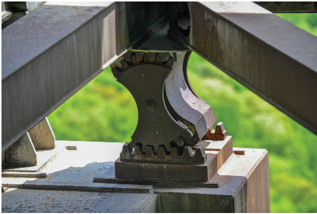
Figure 2.14 Rocker support of the New River Gorge Bridge in West Virginia
