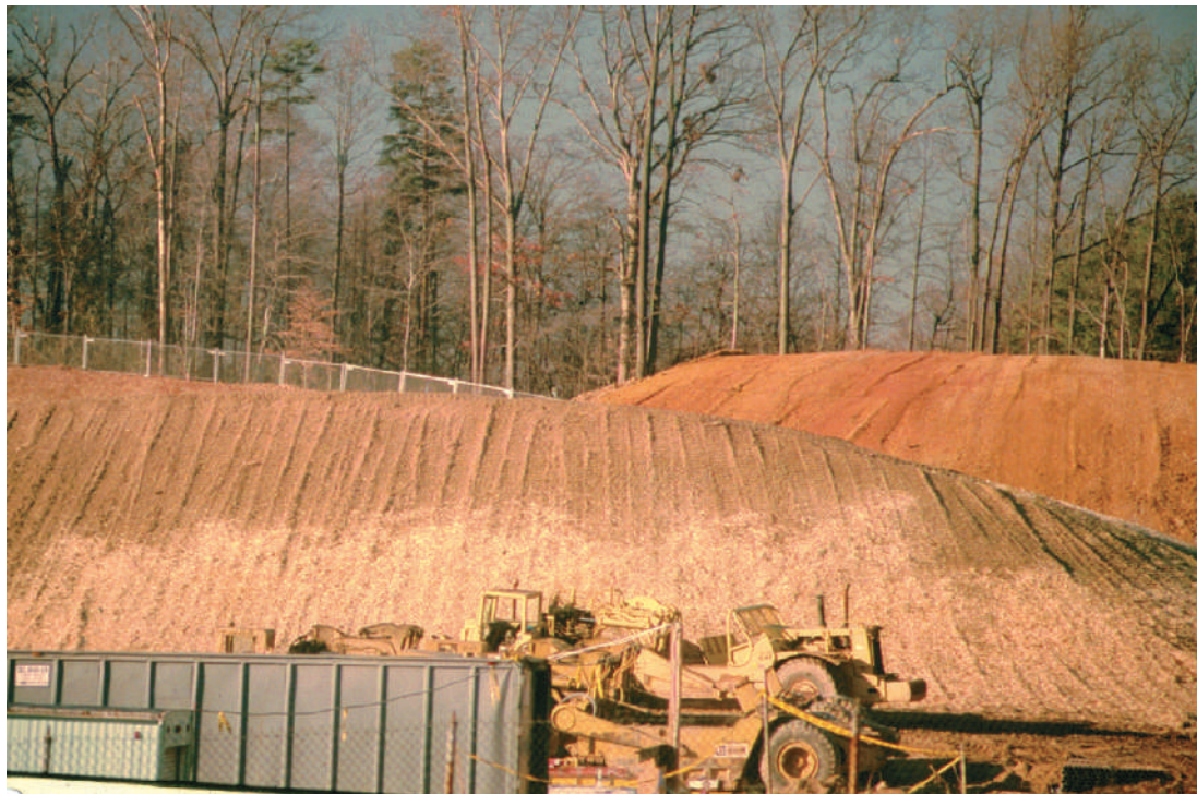
Figure 1.19 The large gray-brown mound of material in the foreground at this construction site consists of topsoil (A horizon material) carefully separated from the lower horizons and pushed aside during initial grading operations. Behind it is a similar sized pile of reddish-brown soil from the lower (subsoil) horizons. The stockpiles were then seeded with grasses to protect from erosion. The subsoil material will be used during construction to fill in low spots and build foundations and roadbeds. After construction activities are complete, the stockpiled topsoil (front pile) will be used in landscaping the grounds around the new buildings. (Photo courtesy of Ray R. Weil)
