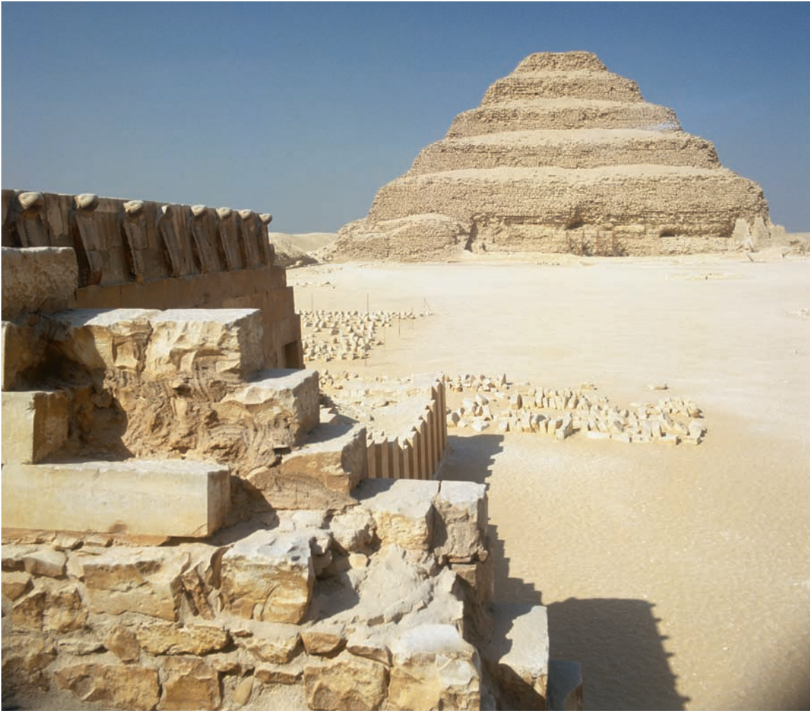
DJOSER'S STEP PYRAMID Djoser ascended to the throne of Egypt around 2668 B.C.E. and immediately ordered his vizier Imhotep to oversee the construction of his tomb. Up until this point, Egyptians constructed pyramids out of mud-brick, but Imhotep deviated from tradition and chose stone.
