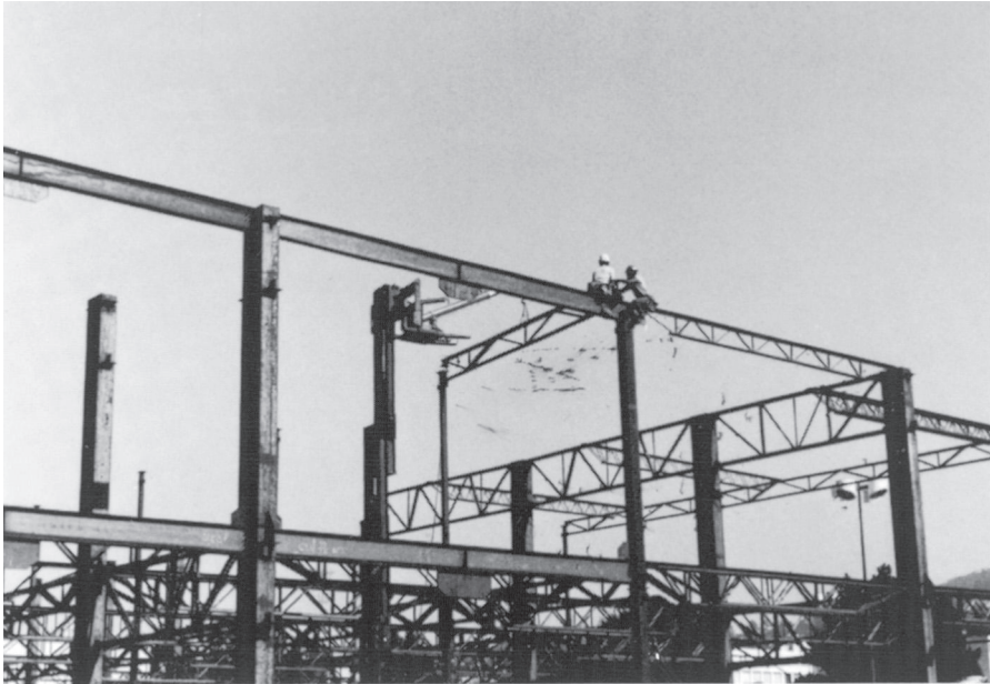
Erection of steel joists. (Courtesy of Nucor Vulcraft Verco Group.)
