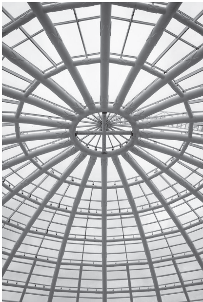
Circular dome steel framed roof system. (Ruslan Gilmanshin/123RF.)
