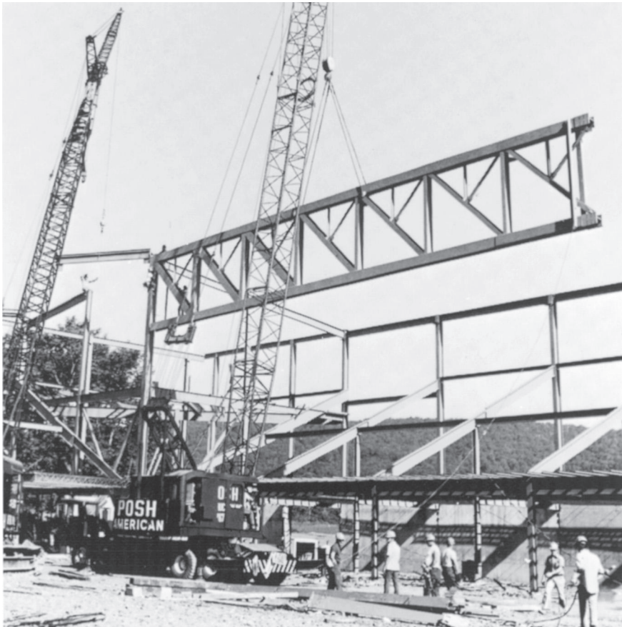
One-half of a 170-ft clear span roof truss for the Athletic and Convention Center, Lehigh University, Bethlehem, PA. (Courtesy of National Museum of Industrial History.)
