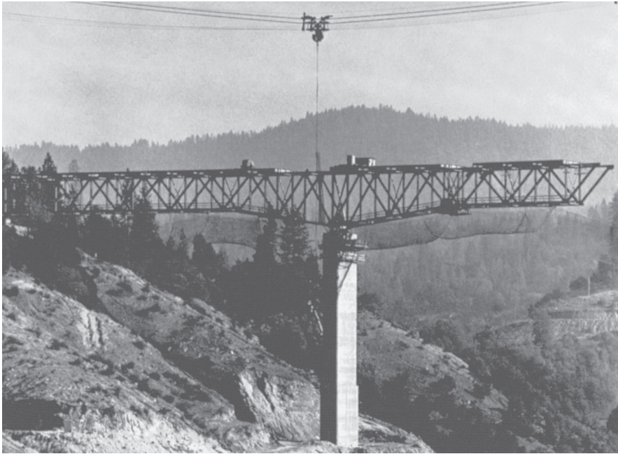
South Fork Feather River Bridge in northern California, being erected by use of a 1626-ft-long cableway strung from 210-ft-high masts anchored on each side of the canyon. (Courtesy of National Museum of Industrial History.)
