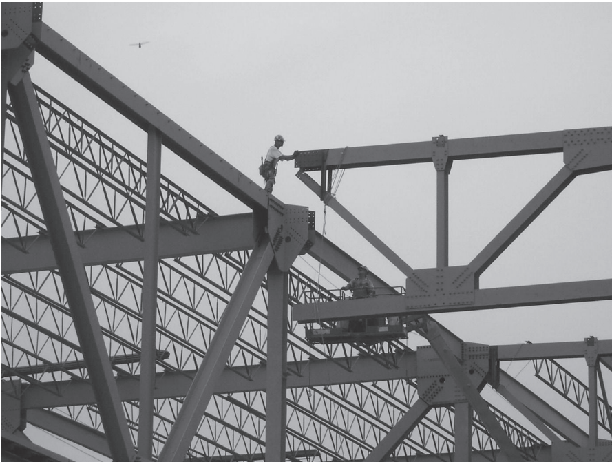
Erection of roof truss, North Charleston, SC. (Courtesy of CMC South Carolina Steel.)
