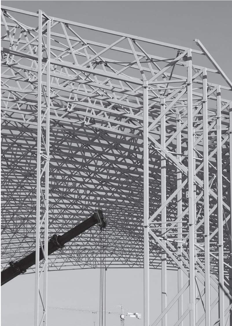
Long span steel framing for industrial building during construction. (Vladimir Prizemlin/123RF.)
