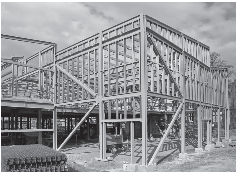
Steel framed commercial building with single diagonal lateral bracing. (stocksolutions/123RF.)
