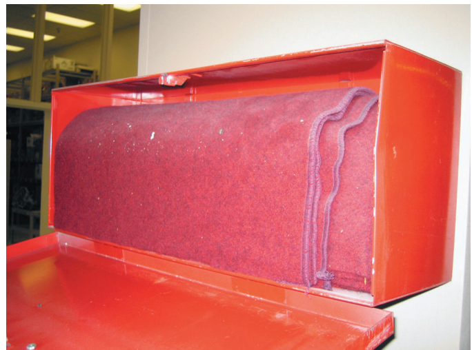
FIGURE 1-81 A treated wool blanket is kept in an easy-to-open wall-mounted holder and should be placed in a central location in the shop.
