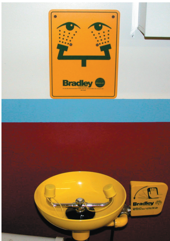
FIGURE 1-83 A typical eye wash station. Often a thorough flushing of the eyes with water is the first and often the best treatment in the event of eye contamination.
