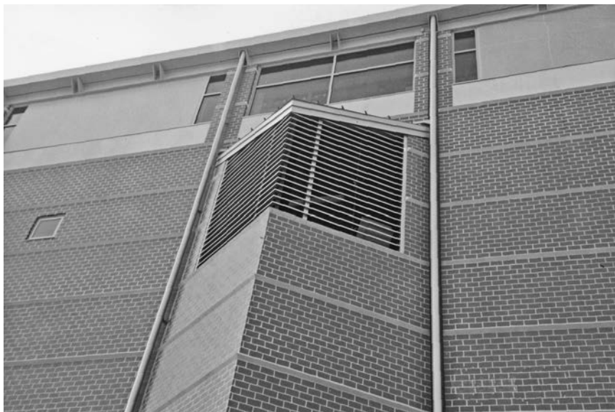
FIGURE 1.6. Air intakes for Monsanto Research Center in St. Louis are placed high to avoid street-level air pollution as a measure to improve indoor air quality.
