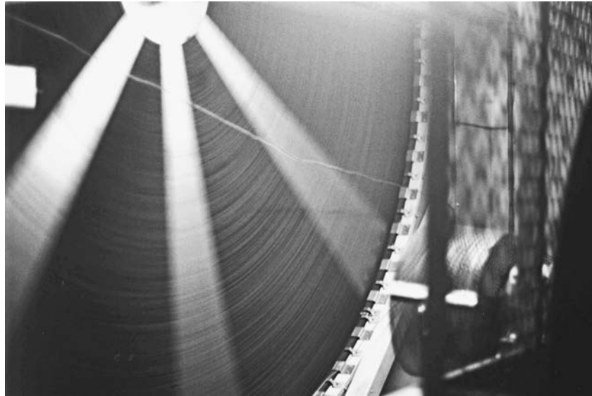
FIGURE 1.5. Heat recovery wheel allows higher ventilation rates without sacrificing economy of operation, exemplifying sustainable design within economic realities.
