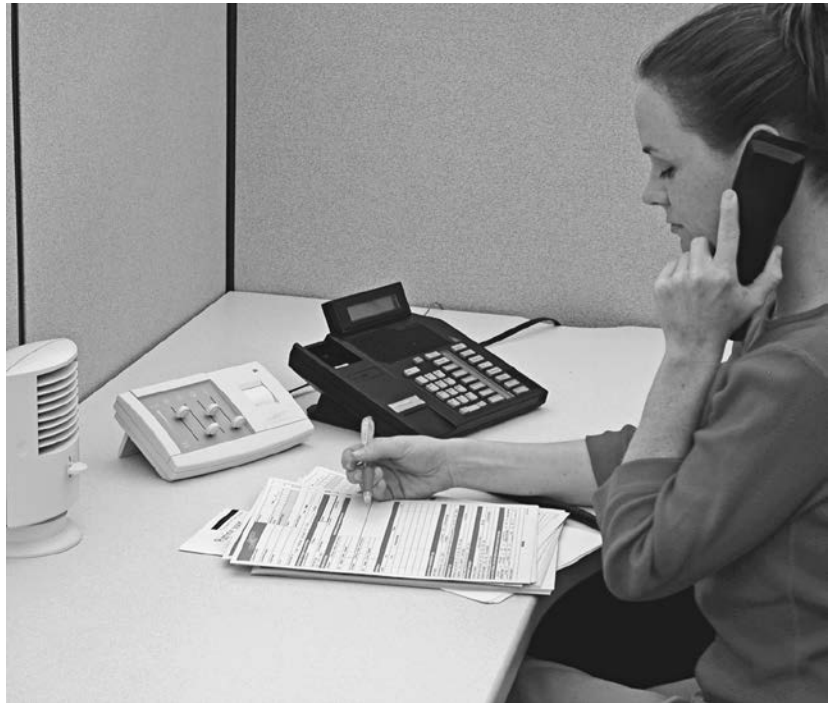
FIGURE 1.7. Personal cooling outlet (left) gives individual personnel control of climate at workstation.
