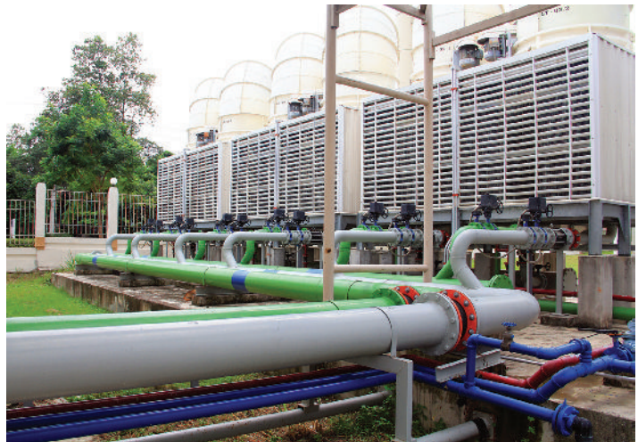
FIGURE 1.1 Complex industrial and commercial fluid piping systems, often unnoticed but critical in our daily lives, require careful design and analysis. The system shown here is required to maintain comfortable temperatures in a commercial building. (Source: Tinnarat Suwanna/123RF)
