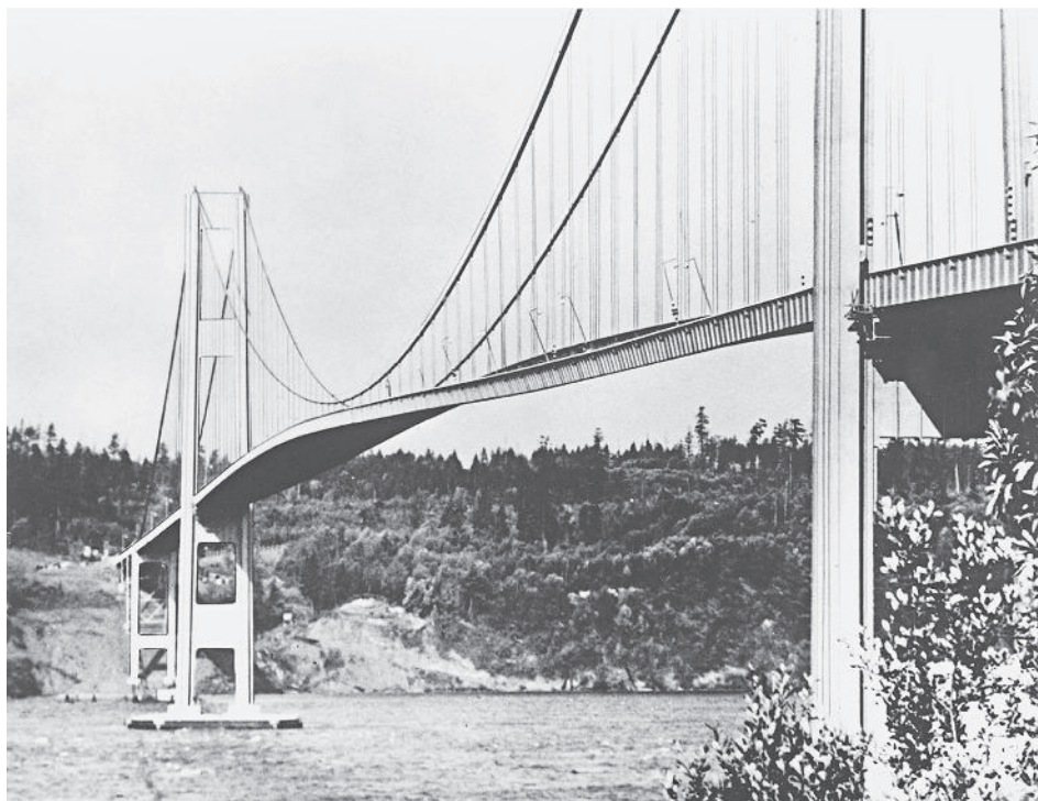
Figure 1.3 The Tacoma Narrows Bridge twisting in the wind. (AP Images)
