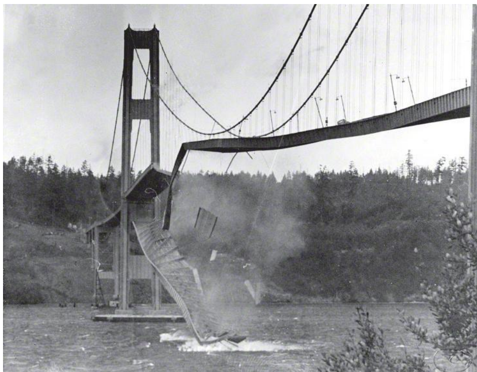
Figure 1.4 The center span of the Tacoma Narrows Bridge plunges into Puget Sound. (AP Images)
