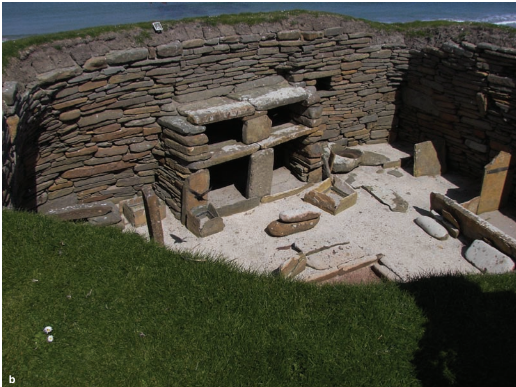
Figure 1.2-8 Orkney Islands, Scotland. Skara Brae, ca. 3000 BCE. (a) Plan, showing (1) thick walls built of dry-wall masonry, (2) individual lodgings featuring built-in furnishings made from stone slabs, and (3) narrow paths connecting the dwellings as a community. (b) Dry-wall masonry from brick-sized stones.
