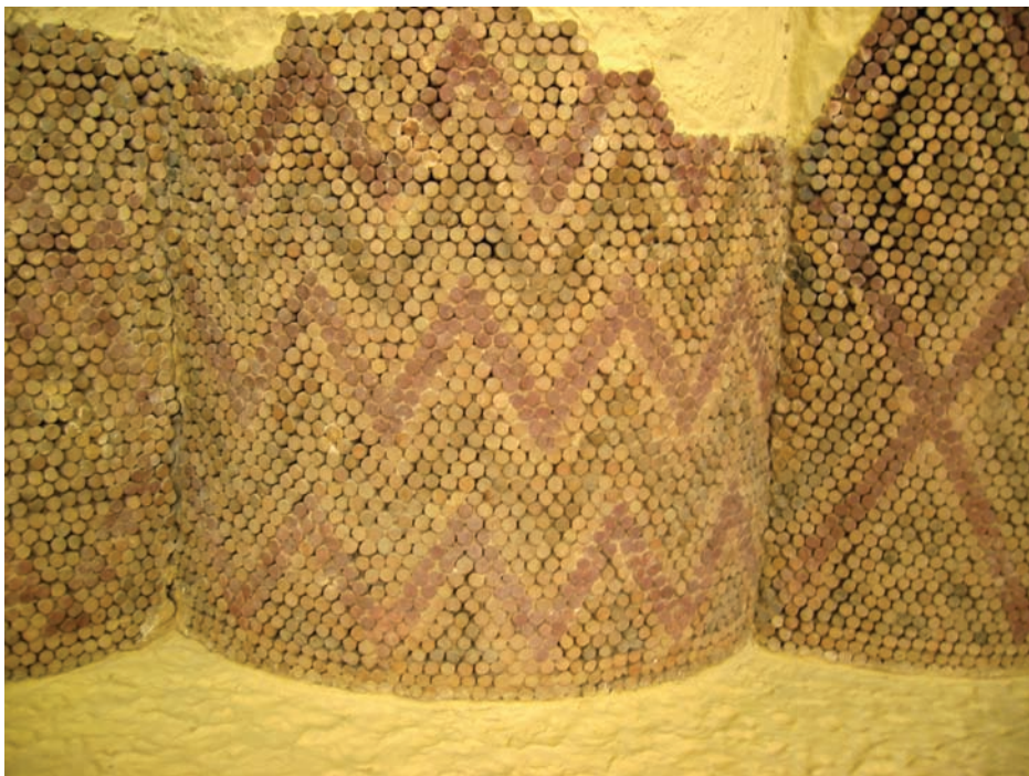
Figure 2.1-5 Uruk, Mesopotamia (Iraq). Cone mosaics covering urban temples with more permanent cladding, ca. 3400–3000 BCE.
