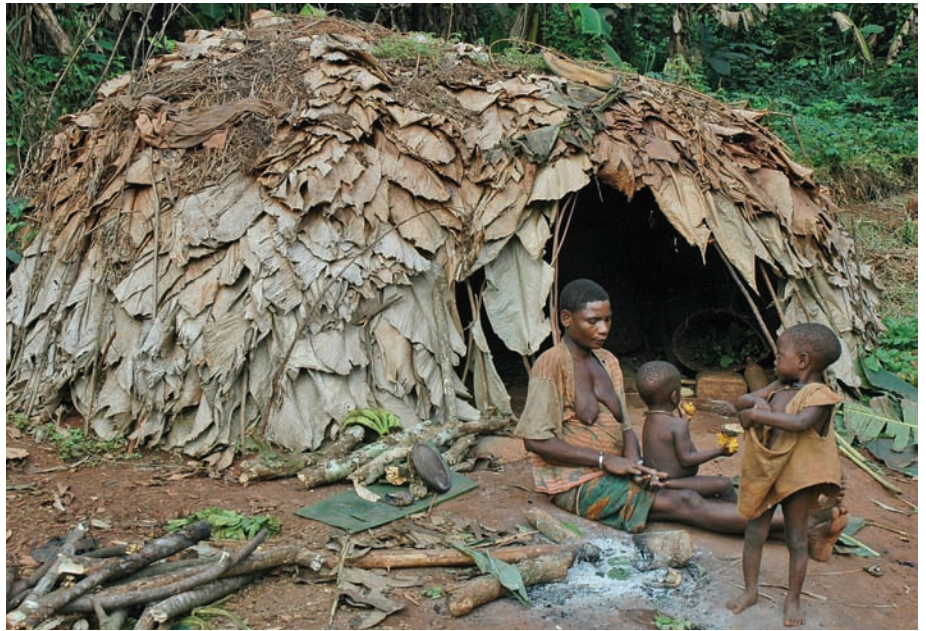
Figure 1.2-1 Cameroon. Baka hut, or mongulu , a semidome of woven branches, covered in mongongo leaves.
