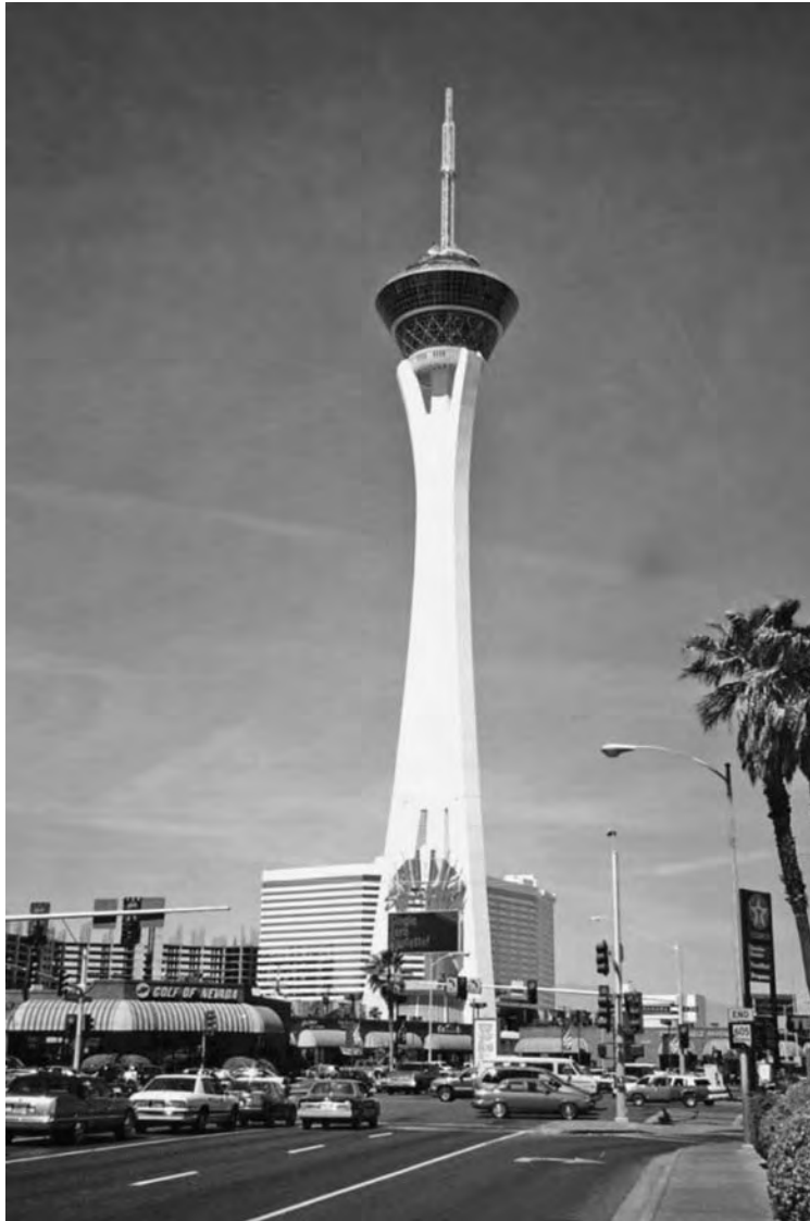
Stratosphere Tower, Las Vegas; the tallest free-standing observation tower in the United States, 1149 feet high. A three-legged concrete tower is topped by a ring beam that supports the steel dome, completed in 1996 (Photo by C. G. Salmon).
