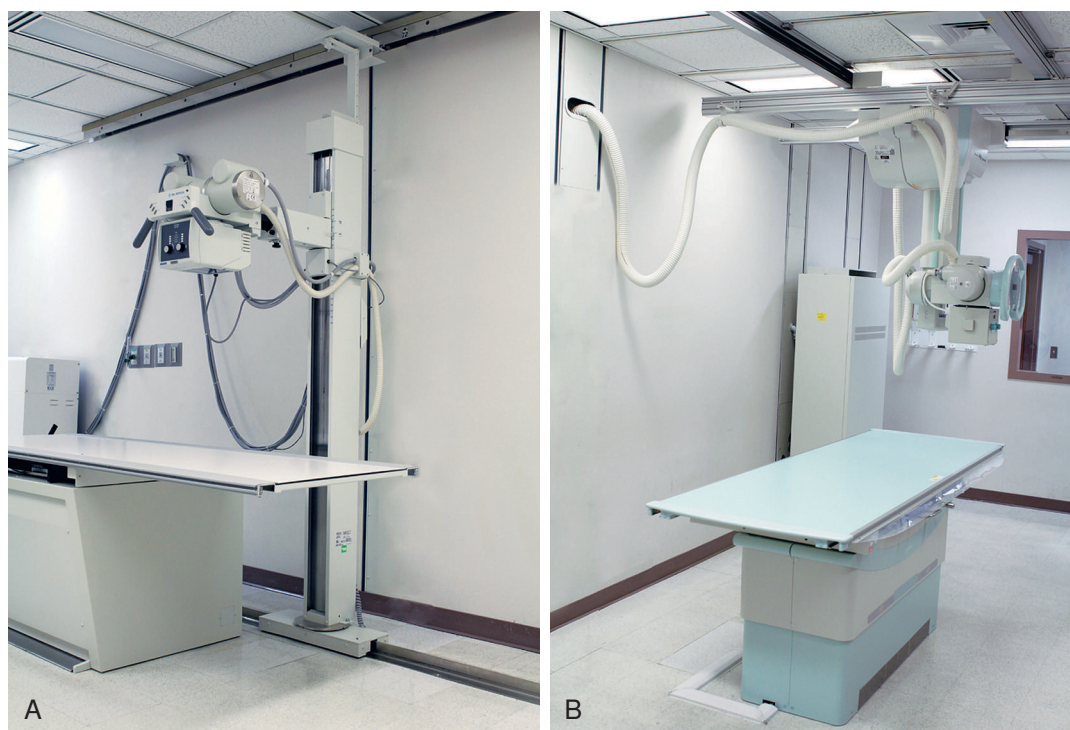
Fig. 1.9 Tube Mount Variations. (A) A floor-ceiling mount. Note the rails along the floor and ceiling. (B) An overhead tube assembly with ceiling-only rails and a telescoping tube crane. This is the most versatile of such designs.
