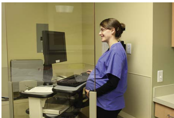
Fig. 3.5 The lead barrier of the control booth protects a pregnant radiographer.
