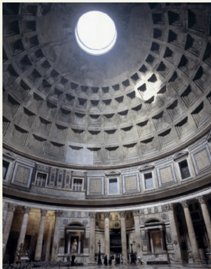
Roman dome with oculus (Pantheon, Rome, Italy, 118–125)
