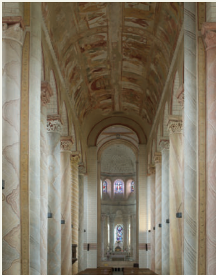
Medieval barrel-vaulted church (Saint-Savin, Saint-Savin-sur-Gartempe, France, ca. 1100)
