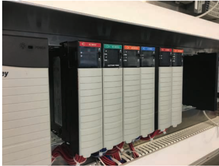
Figure 1–4 PLC Chassis with I/O Modules Installed
