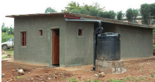
FIGURE 1.16 Completed model home in Rwanda made from earth-block construction with a rainwater harvesting system shown in the foreground that is sitting on top of the visible portion of an underground biogas digester.
