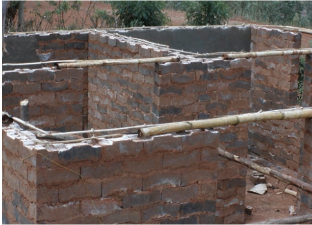
FIGURE 1.15 Interlocked earth-block construction methods use inexpensive soil-based construction blocks that are made primarily from materials available near the construction site and use locally harvested bamboo reinforcement for construction.
