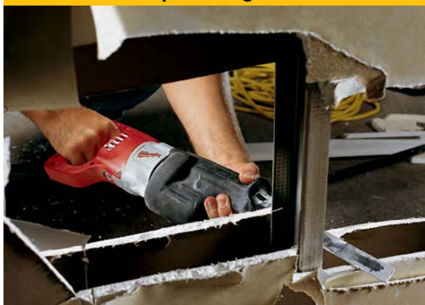
Figure 2-21. Reciprocating saws are used by industrial and mechanical technicians to make cuts into finished walls, ceilings, and floors.
