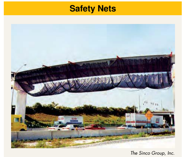
Figure 1-17. A safety net must be installed whenever a worker is 25' or more above the ground, water, machinery, or other solid surfaces when technicians are not otherwise protected by fall-protection equipment or guardrails.
