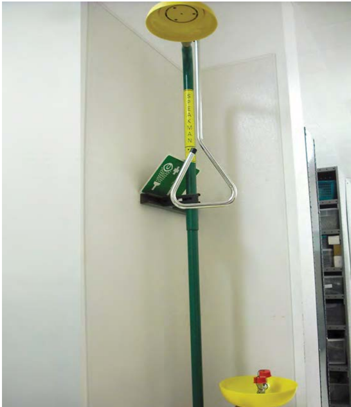
Emergency eyewash stations and deluge shower units are used to flush chemicals and other contaminants from the eyes and body and provide first aid to burn victims.
