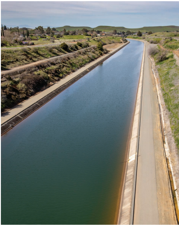
Figure 1.6 Key component of California's vast State Water Project. One of the largest of its kind in the world, the project collects water from the state's northern watersheds and redistributes it to more arid zones in the southern part of the state, using a network of 21 dams and more than 700 miles of canals, tunnels, and pipelines. Although about 70% of the project's water goes to urban and industrial uses, it is connected to and forms an important part of other water systems in the state that primarily provide irrigation water to farms. Systems such as this have dramatically altered streams and hydrologic function.
