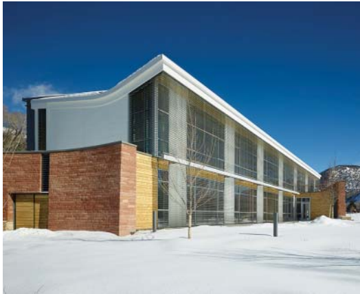
Fig. 1.24 South façade showing solar shading devices and daylight apertures. (Courtesy of ZGF Architects LLP; © Tim Griffith.)
