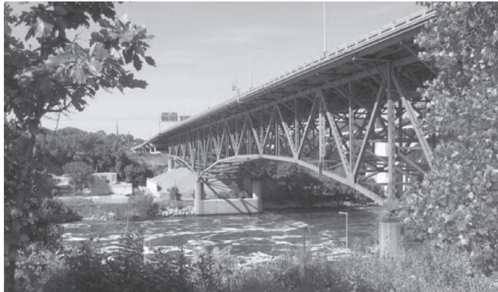
Fig. 2.14 Center span of I-35W bridge looking northeast. The center span is supported by pier 6 on the near (south) riverbank and pier 7 on the far (north) riverbank. (NTSB, 2008).
