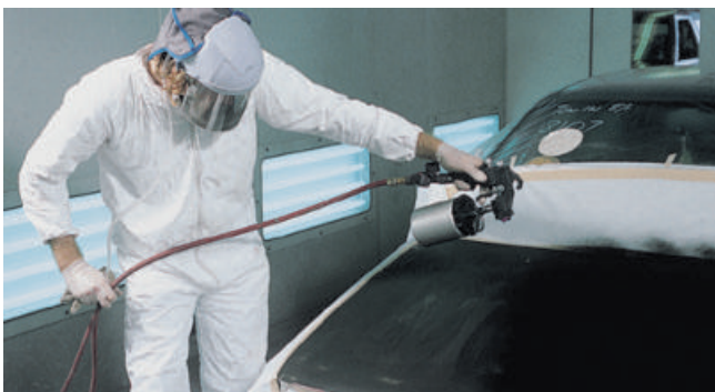
Figure 1-29 Excellent hand-eye coordination and specialized knowledge is needed to be a professional painter. (A) When painting a vehicle, keep the gun the correct distance from the surface. Also keep the gun parallel with the surface. (B) When painting, try to move the spray gun smoothly and evenly. Use straight line paint strokes that overlap evenly. If you move the gun at different speeds or move it further or closer to the surface, paint problems will result.
