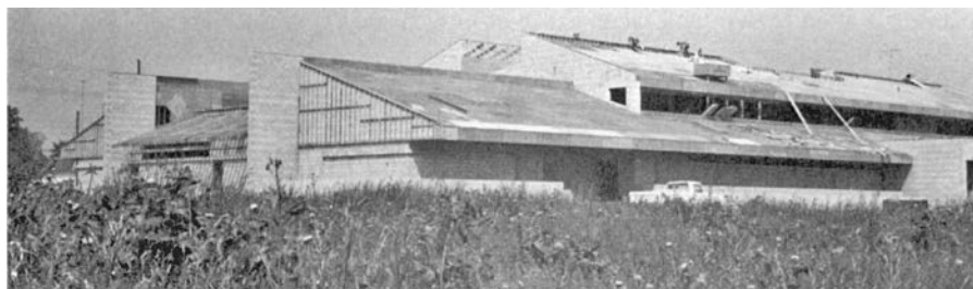
FIGURE 1.2B Building with reinforced-masonry block walls and a wood roof system with plywood sheathing. (Photo courtesy of Mark Williams.)
