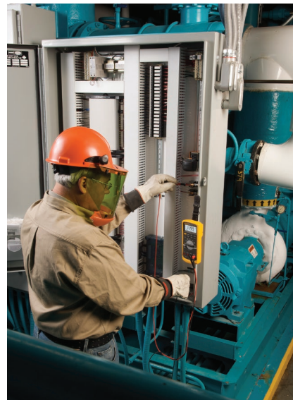
Figure 1-18 Testing for the presence of voltage.
