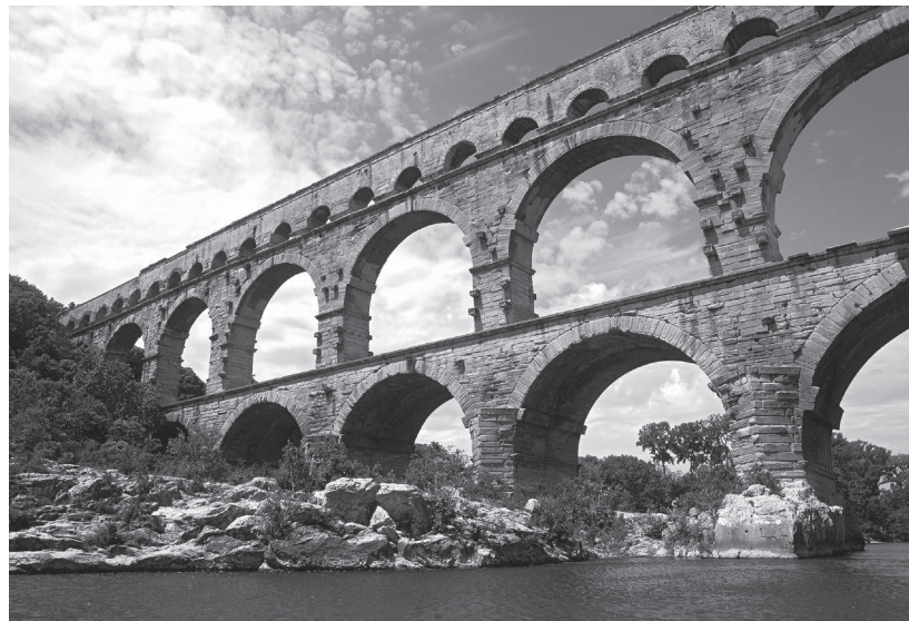
Photo 1.2: Romans pioneered in the use of arches for bridges, buildings, and aqueducts. Pont-du-Gard. Roman aqueduct built in 19 B.C. to carry water across the Gardon Valley to Nîmes. Spans of the first- and second-level arches are 53 to 80 ft. (Near Remoulins, France.) Apply Pictures/Alamy
