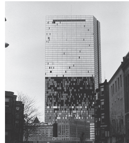
Photo 1.1: Wind damage. Shortly after thermopane windows were installed in this high-rise office building, they began failing and falling out, scattering broken glass on passers-by beneath.
