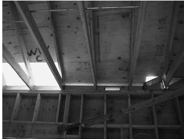
FIGURE 1.4 Photo of incomplete load path—blocking issue.
