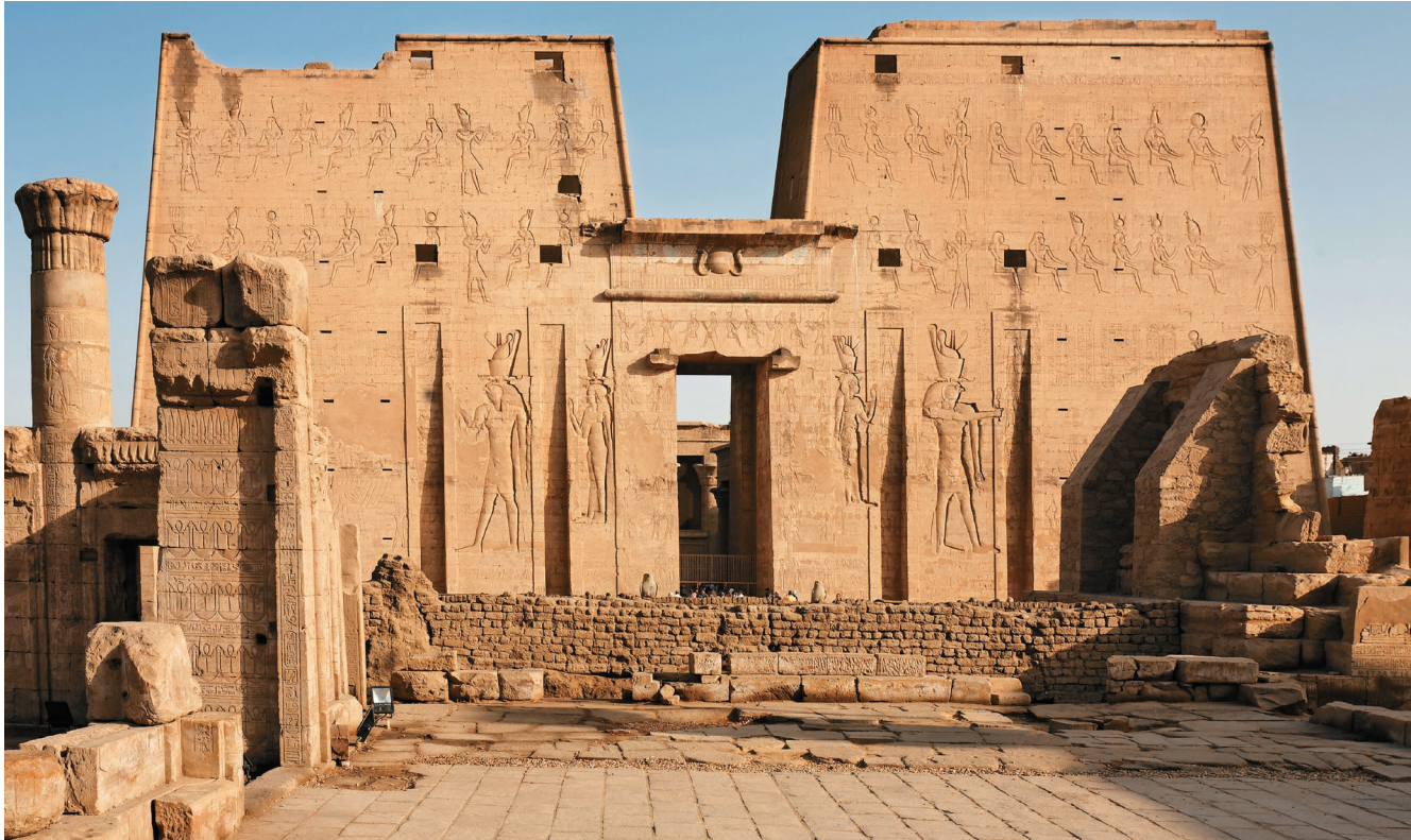
1.32 (above) Pylon gateway, Temple of Edfu, Egypt, 237–57 BCE. While this pylon dates from the Ptolemaic period after Alexander the Great conquered Egypt, it is similar in form and purpose to those at Karnak. Such a spatial threshold signified the increasing sacredness of the space beyond. The four vertical slots once held obelisks. Ostili/Getty Images
