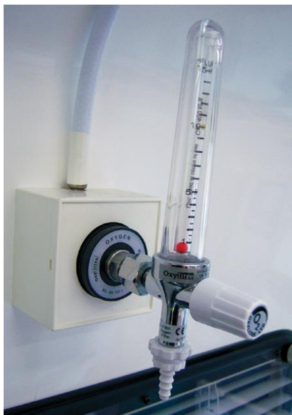
FIGURE 1-7 Oxygen and air DISS connections to an oxygen flowmeter.
