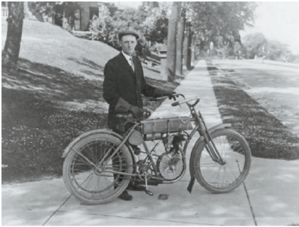
Figure 1-12 The first V-Twin built by Harley-Davidson had 7 horsepower and was built in 1909.
