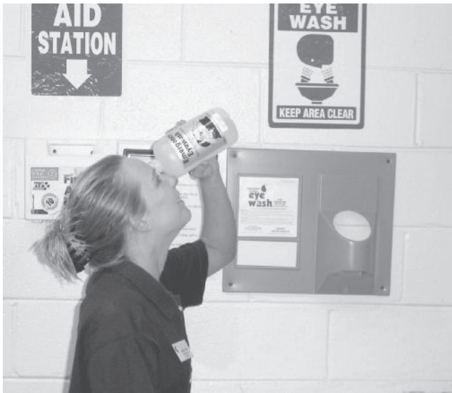
Figure 2-12 Eye-wash stations are available in properly equipped motorcycle service shops. If you need to use an eye-wash station, you should follow up with a visit to a doctor to ensure no permanent damage to the eyes has occurred.
