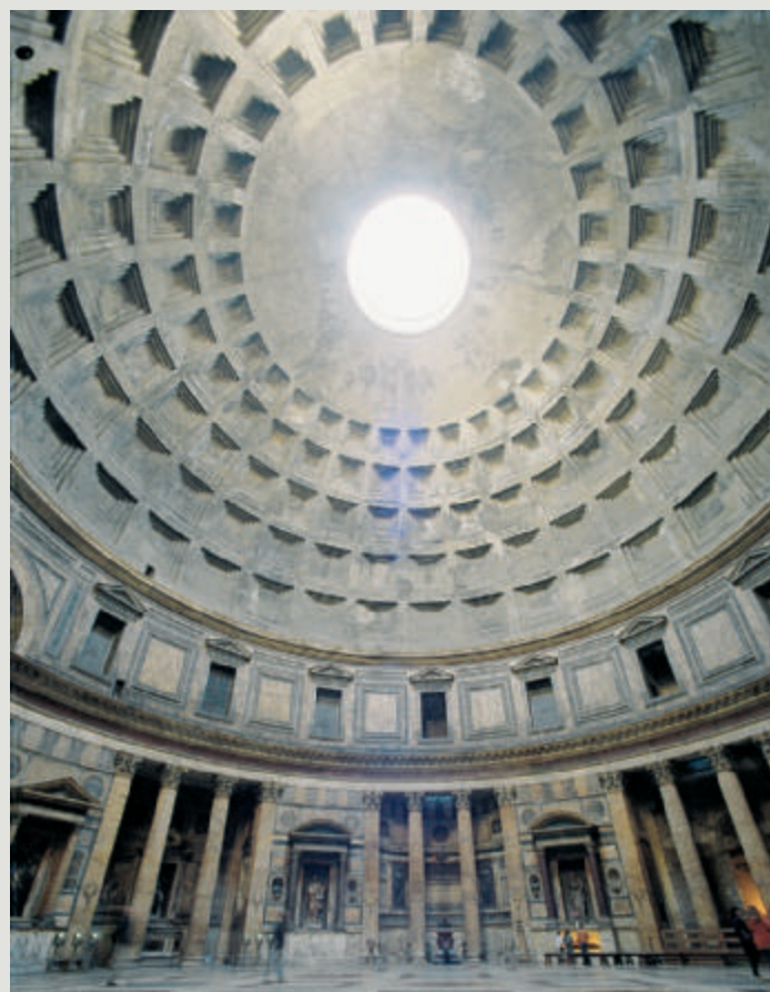
Roman dome with oculus (Pantheon, Rome, Italy, 118–125)
