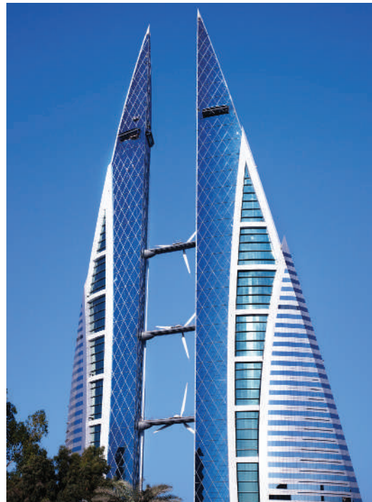
FIGURE 1.5 Once the architectural team has designed a structure, the engineering team is responsible for determining the loads that a structure must resist and ensuring that those loads are transferred to the foundation and into the supporting ground. Engineers working on this structure in Manama, Bahrain, not only had to plan for the normal loads of a structure, but they also had to design the structure in such a way that the twin 50-story towers would support the three wind turbines that are used to help supply energy for the structure. © Yoshio Tomii/The Image Bank/Getty Images.
