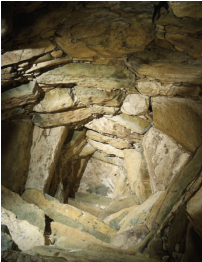
1-17 Corbeled dome of the main chamber in the passage grave, Newgrange, Ireland, ca. 3200–2500 BCE.
