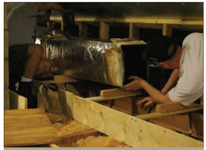
FIGURE I-12 Duct insulation increases system energy efficiency.
