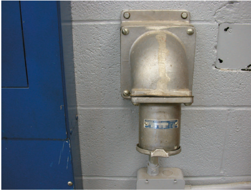
FIGURE 1–11 High-voltage three-phase electrical outlet.
