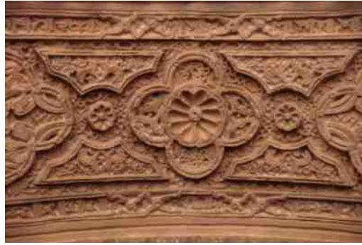
FIGURE 1.22 Band patterns use repeated single or multiple motifs and are found on moldings, frames, linear forms, and around columns.
