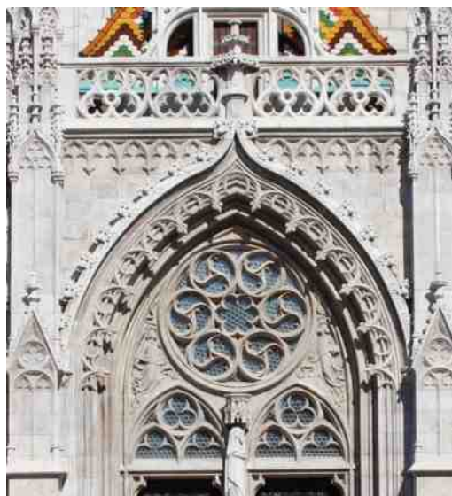
FIGURE 1.24 A number of geometric forms are employed on this entry, although the ogee arch formed by elongated S-curves dominates.
