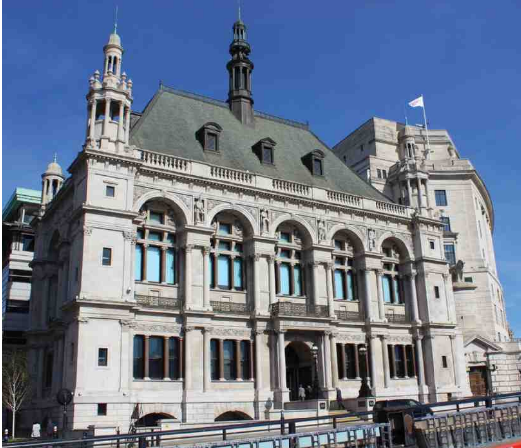
FIGURE 1.4 Engaged columns may be a part of the wall structure of a building, projecting outward from a few inches to almost their entire diameters.
