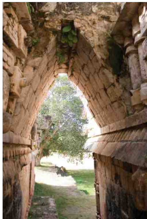
FIGURE 1.2 The earliest cantilevers were used to roof buildings, with each successive horizontal layer projecting slightly beyond the one beneath it until the two sides met at the top.
