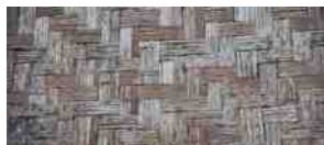
FIGURE 1.8 In tropical areas, buildings often employ walls or roofs made of vegetative materials that breathe.
