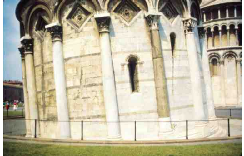
FIGURE 1.6 The Leaning Tower of Pisa, started in the eleventh century, began to lean during construction. Rather than abandon it, architects tried to compensate for the lean by raising the height of one side of successive layers.
