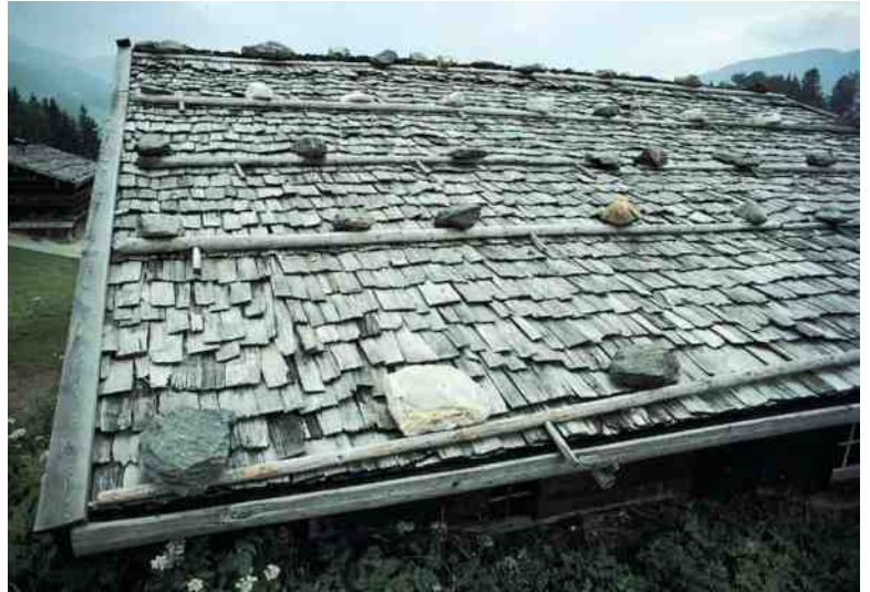
FIGURE 1.9 Snow is an excellent insulator, and Swiss roofs may have low fences or stones to retain snow on the roof for that purpose.
