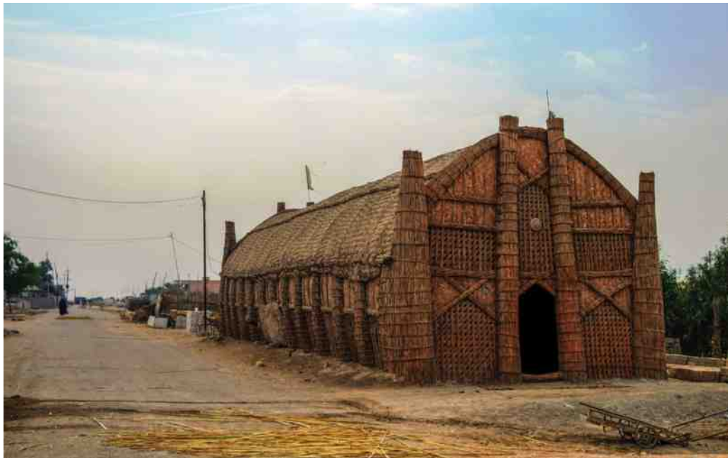
FIGURE 2.3 Modern houses in the marshes of Iraq are strikingly similar to the reed structures depicted in ancient drawings and reliefs. Bundles of reeds are tied together to form a framework. Reed mats or wattle and daub may fill the spaces between the bundles.
